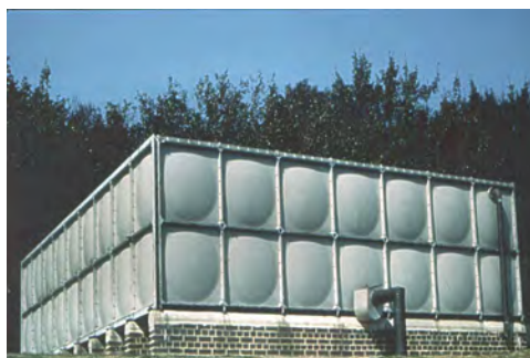
Above: water tank panels in SMC used for their freedom from corrosion and low maintenance
