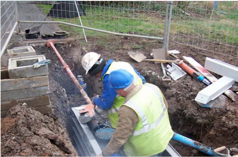
SMC underground junction box. These modular boxes are used to replace brick chambers built in-situ, and are used for joining pipes, drains and cables. Good mechanical strength and resistance to acid and alkali attack are essential requirements.
