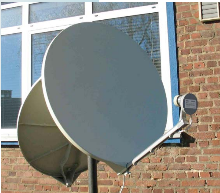
Satellite aerials are frequently made from SMC/BMC.
